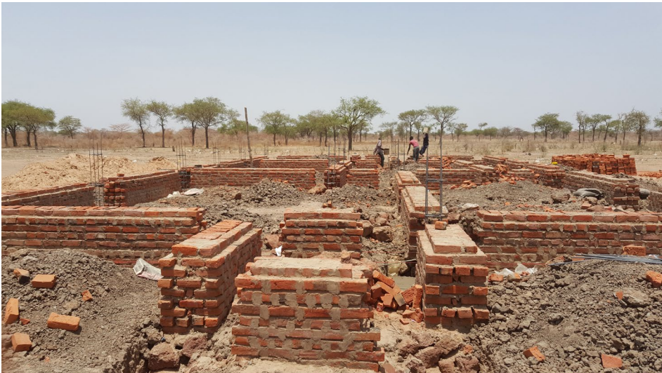
Image 4 New detention centre under construction
