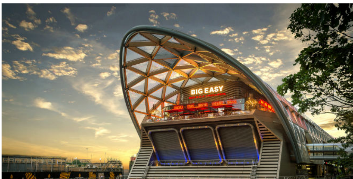
The site of the future Crossrail station at Canary Wharf, London. Photo: Nick Moulds via a CC-BY-NC-SA 2.0 licence
