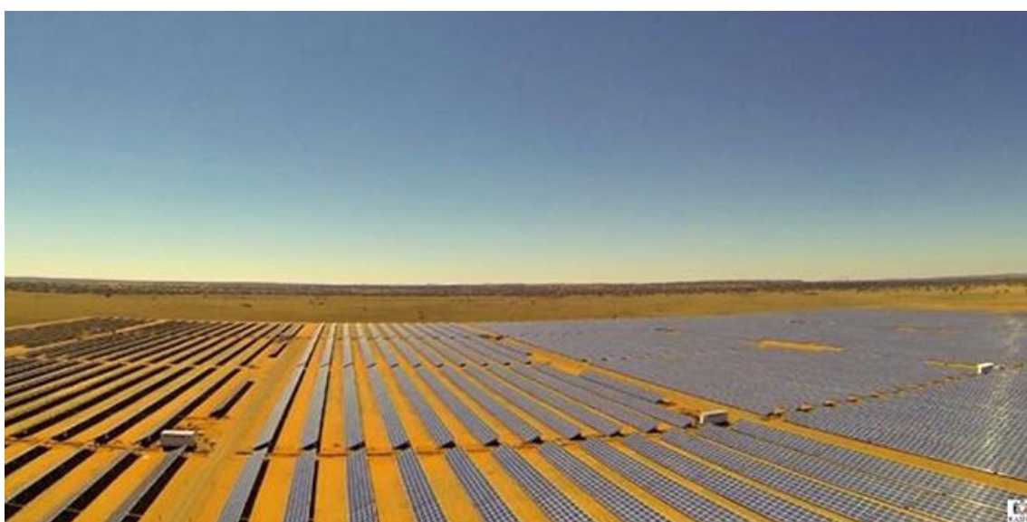
The Droogfontein solar plant near Kimberley opened in 2014 Photo Credit: Kasif Parthan via Flickr ( http://bit.ly/2iHSqvo ) CC BY-SA 2.0
