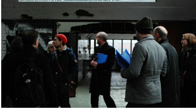
The group sees inside the Grade II listed building that will be converted into a primary school
