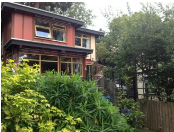
Walter's Way Self-Build Houses
