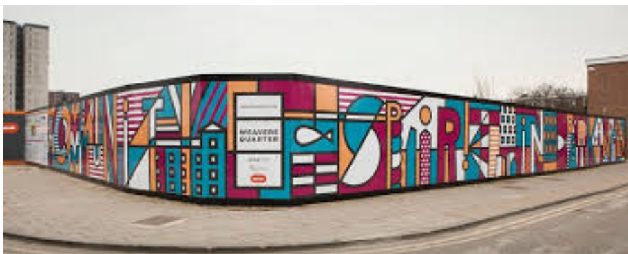
The building works, where flats have been demolished to be replaced by more 'modern' builds. The sign reads 'Weaver's Quarter'.
