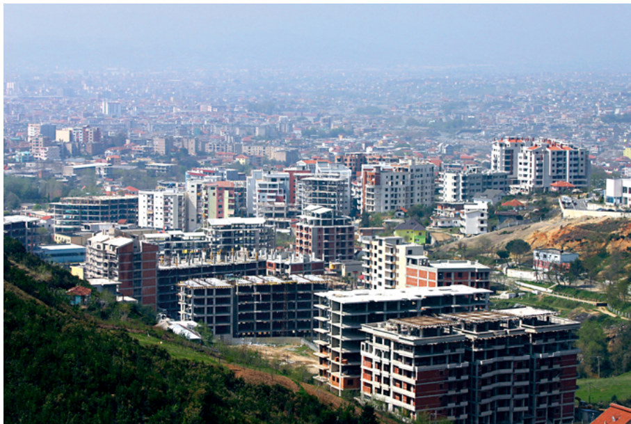
Construction in Tirana. Photo: Gazeta Dita, Albania
