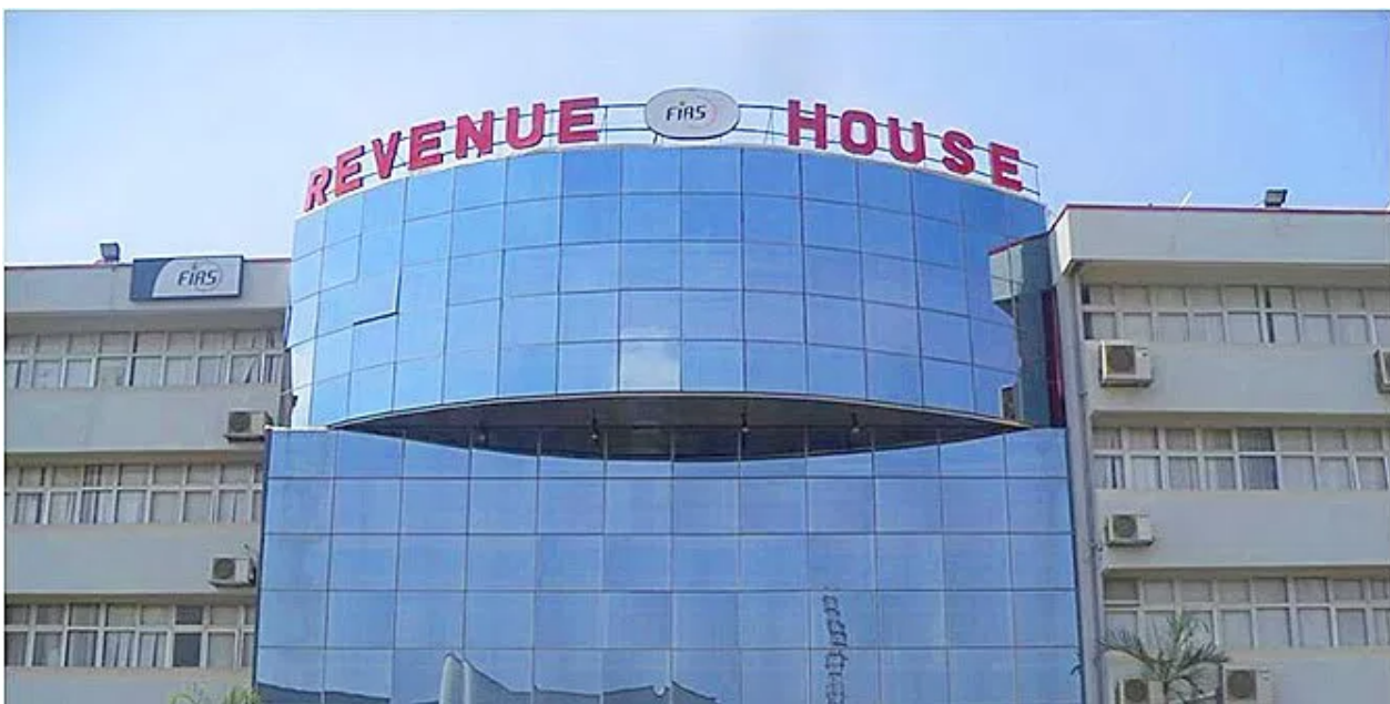
Nigeria Federal Inland Revenue Services (FIRS) building Photo Credit: Lagos Made ( http://bit.ly/2mk4UMp )
