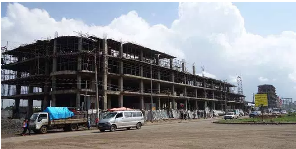
Construction along new road links in Addis Ababa
