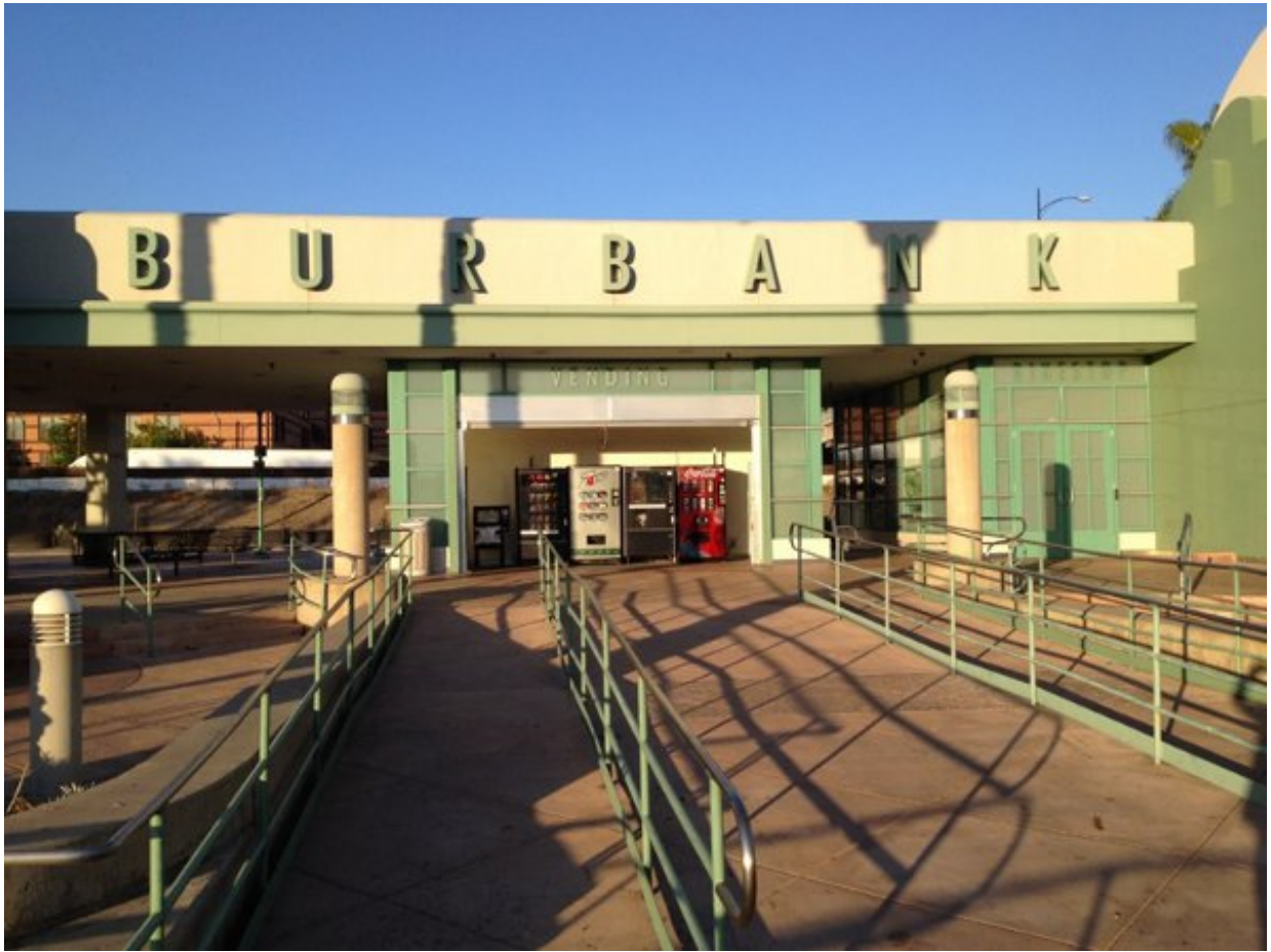
Figure 2 – Burbank Metrolink Station, back view (Golden State Freeway)
