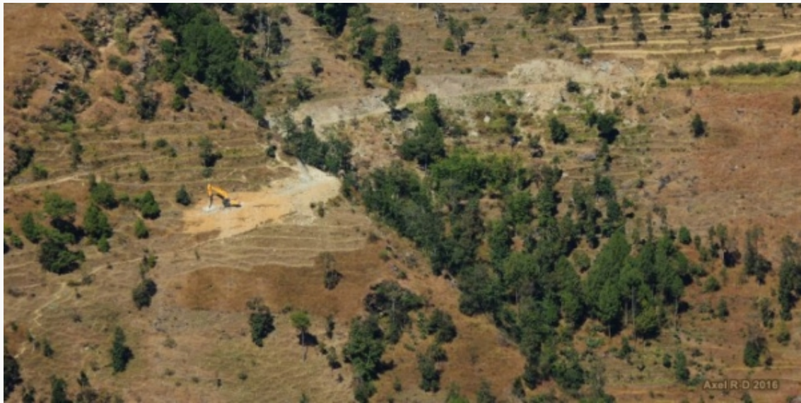
Image: New road in progress. Credit: Axel Drainville CC BY-NC 2.0
