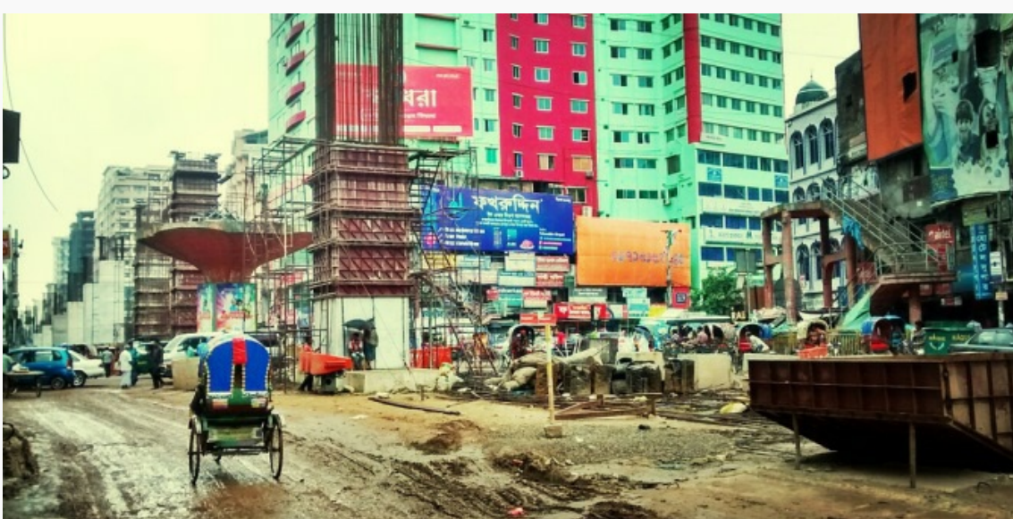
Moghbazar, Dhaka. Cityscapes under construction. Credit: nasir khan CC BY-SA 2.0
