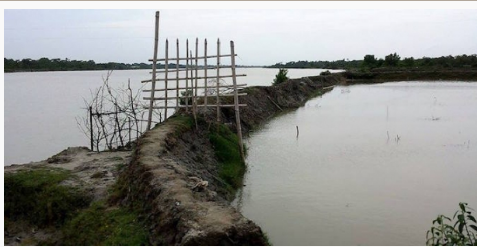
Once a polder embankment is breached, the island becomes waterlogged for months on end. Credit: Meraz Mostafa
