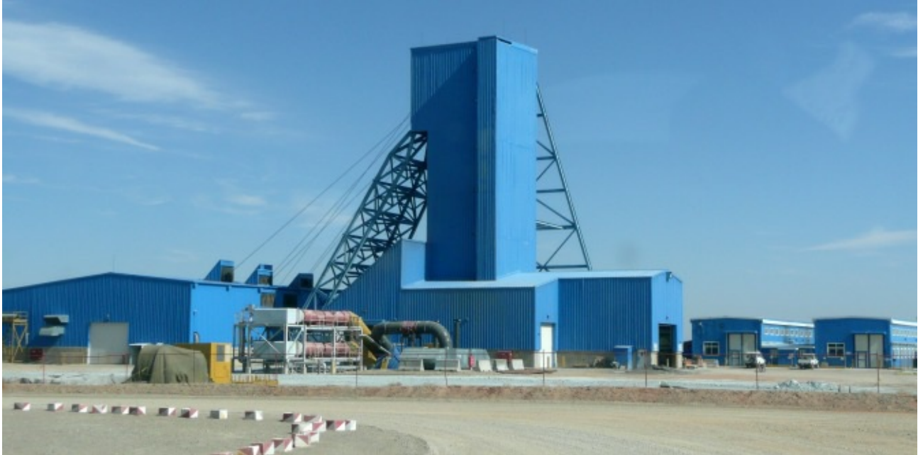
Shaft #1 at Oyu Tolgoi copper mine in Ömnögovi Province, Mongolia, by Brücke-Osteuropa , own work, Wikimedia Commons , Public Domain
