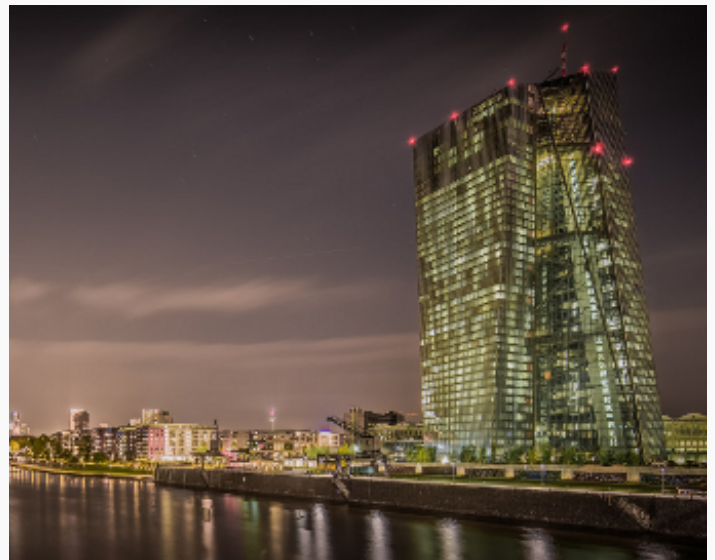
The new ECB headquarters, under construction in Frankfurt, Credit: Frank Friedrichs (CC-BY-SA-3.0)
