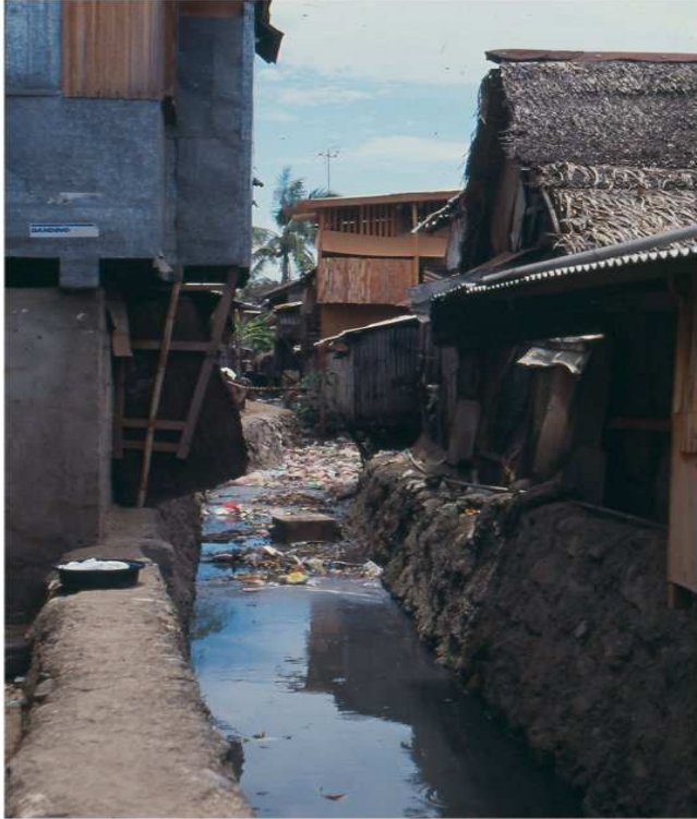
FIGURE 3: OPEN DRAINAGE CHANNEL, CEBU CITY, PHILIPPINES
