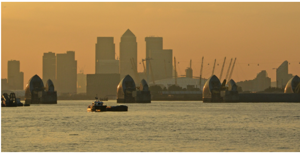
A view of London through the Thames Barrier
