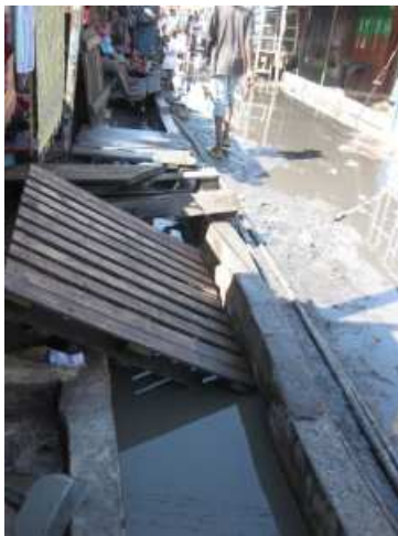
A sewer in Old Fadama, Ghana's largest informal settlement.
