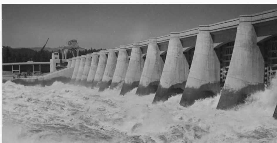
Benneville Power Dam, Columbia River, Oregon. Spillway." US Army Corps of Engineers. Credit: Franklin D. Roosevelt Presidential Library & Museum
