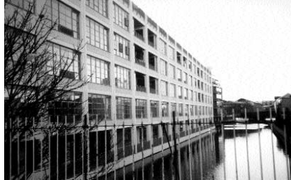
Warehouses are converted to new office buildings in a gentrifying neighbourhood in Inner London.
