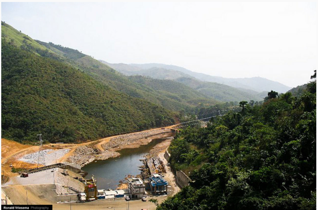
Sierra Leone – Bumbuna Hydro Power station. In Sierra Leone, roughly five percent of people have access to electricity, while those that do have had to acclimate to sporadic blackouts because of the lack of a stable power supply. Credit: Ronald Vriesema CC BY-NC-ND 2.0
