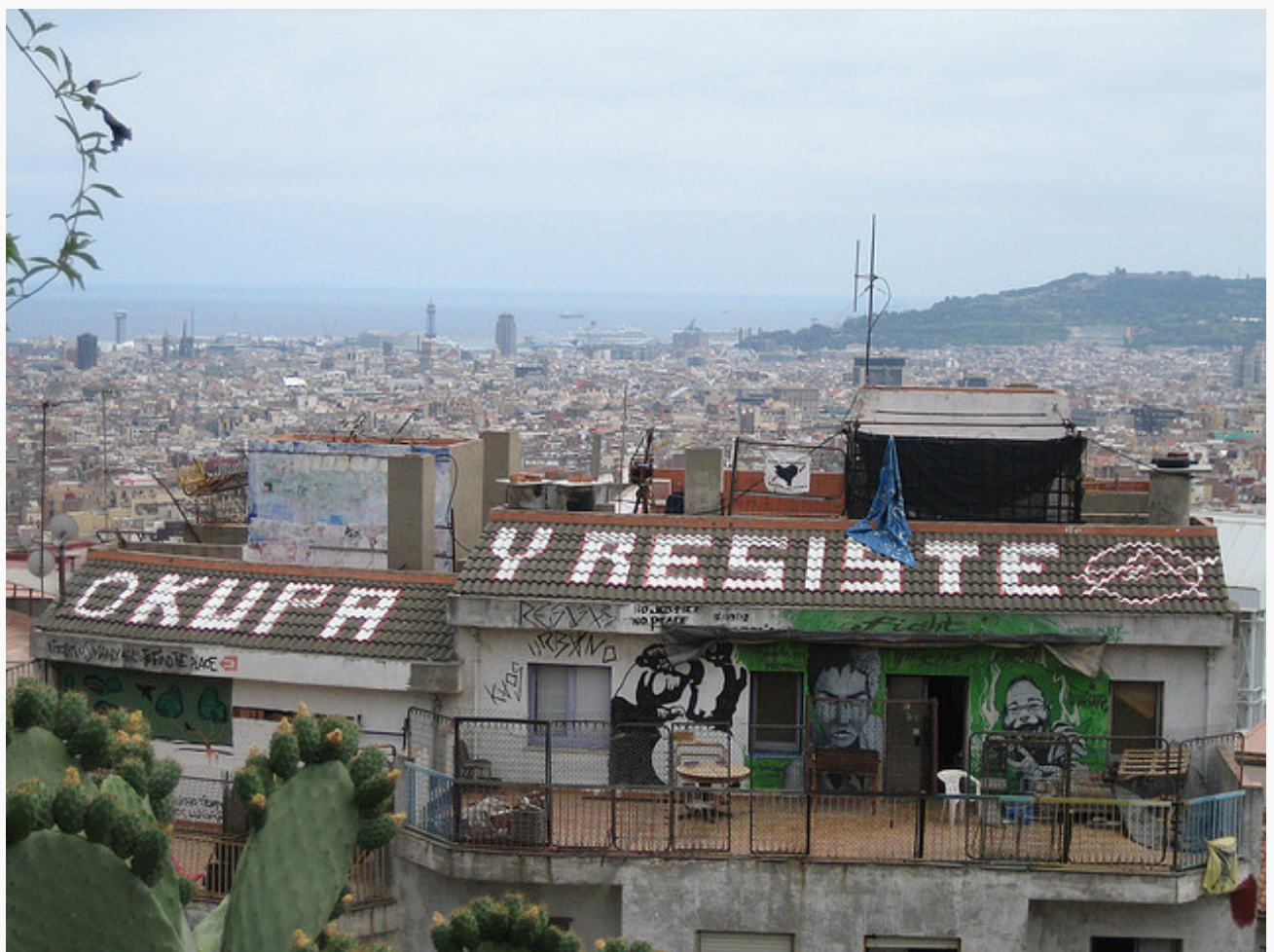
Anarchist building visible from Parc Guell, Barcelona. Credit: jtu CC BY-NC 2.0
