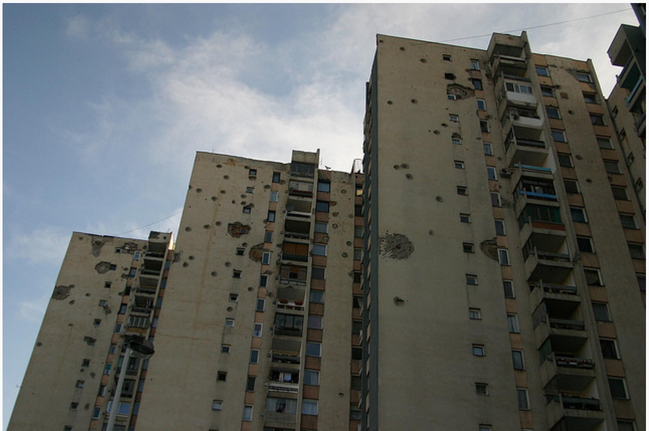
Damaged tower blocks in Sarajevo. Credit: PnP! CC BY-NC-ND 2.0
