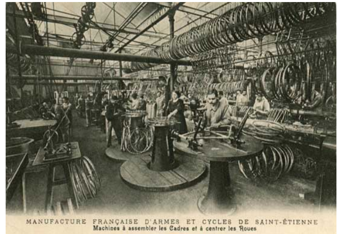
Figure 6: Bicycle frame and wheel assembly at the Manufrance factory
