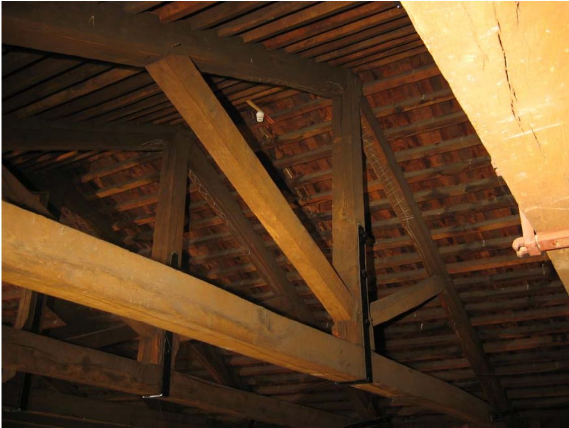
Figure 3. St Paul's Cathedral, roof truss over the nave.
