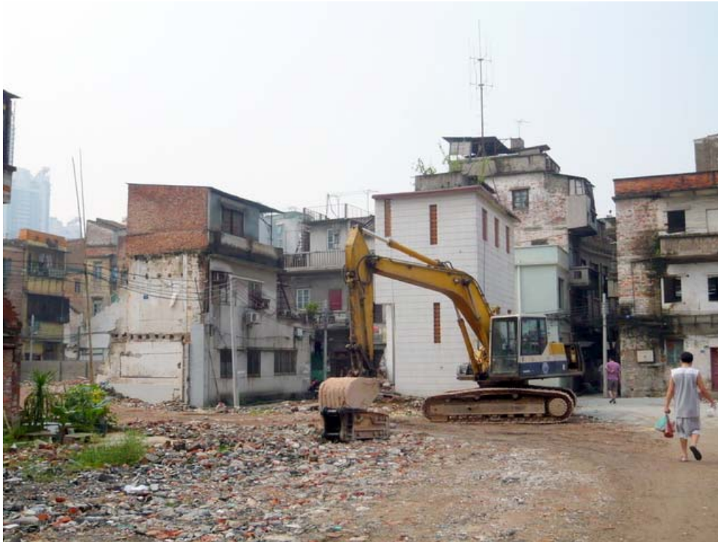
Fig. 12.2 Demolition in progress (near Yuanhe Street) (Author's own picture dated 9 Sept 2010)
