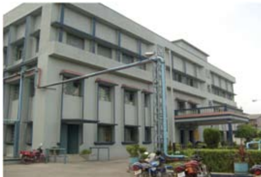
Front entrance to the main building
