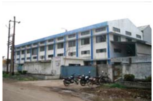
Plant buildings with gates and guard post
