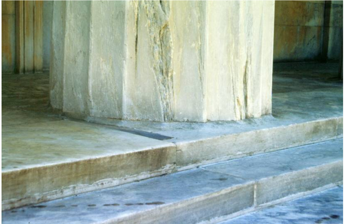
Fig. 22 Philadelphia, PA. Second Bank of the United States. Drum of marble column set on the floor as in antiquity.
