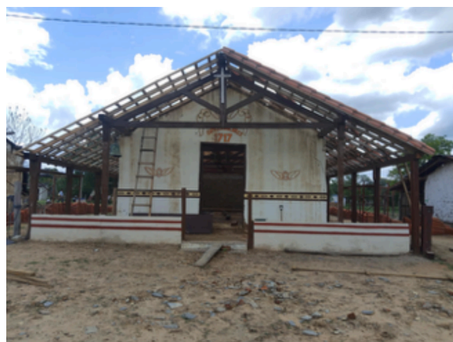
Fig. 10. Project "extension and repair" of the original Jesuit Church, Dolores, Nov 2024.
