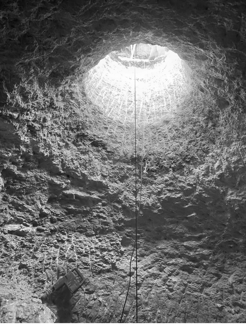
5 The neck of a cistern during its hewing in Wādī Al-'uqda, October, 2021
