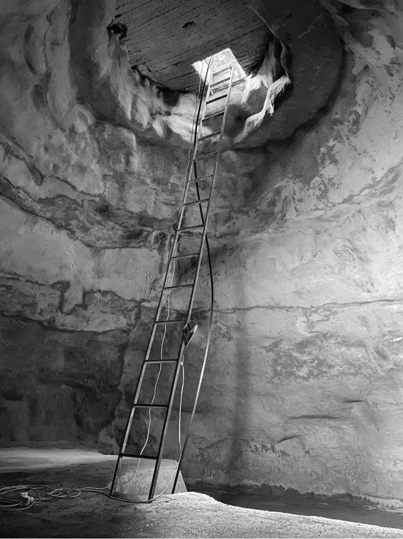
2 Inside an 'injaša cistern during renovation. Ramallah, October 2021
