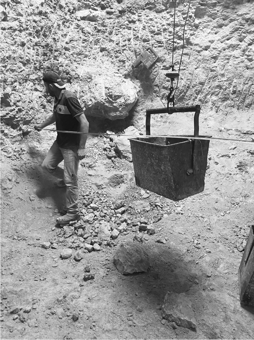
6 Mohammad taking measurements of the cistern during its hewing in Wādī al-'uqda, October, 2021. To his right is his komprīša .
