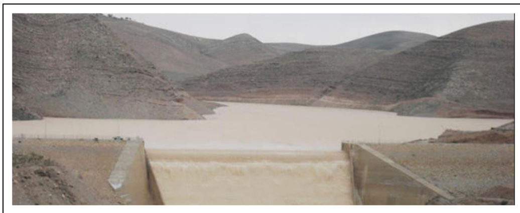
Figure 2. Wala River Dam (Photo by the author).
