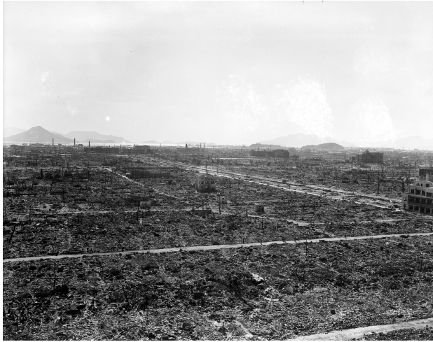
(a) Total destruction near the epicenter
