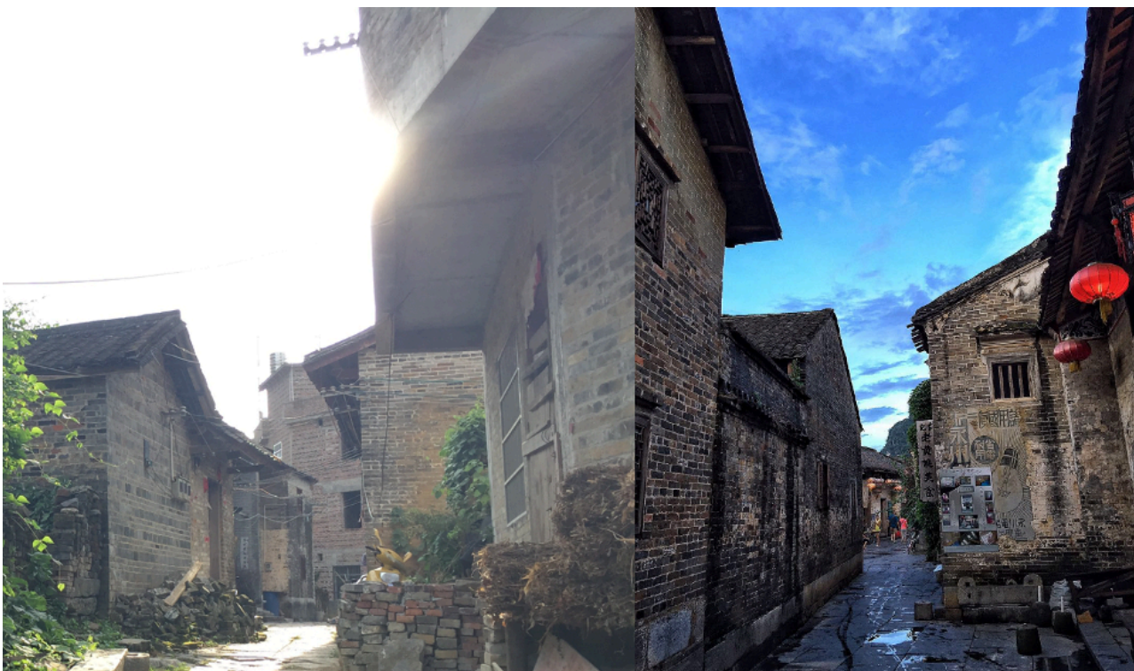
Figure 2. A comparison of the main street side (right) and the backstreet side (left) of where Relevant Hotel stands. Electricity wires can be seen under the eaves and across the backstreet. However, electricity wiring like this should not appear on a main street. Photographed by the author in July 2017
