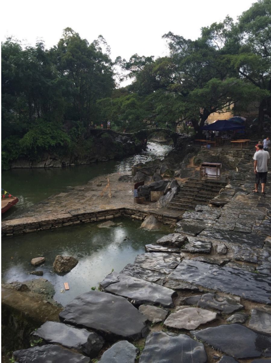
Figure 1. A brooklet and a stone bridge in Huangyao Ancient Town. Nine old streets shape the Ancient Town. All the old streets are paved with green-grey slate. Photographed by the author in July, 2015.
