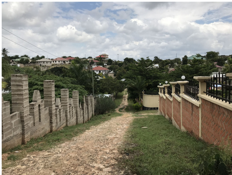
Figure 5: Orderly and well-maintained paths and walls between plots, Salasala July 2018 (photo by author)
