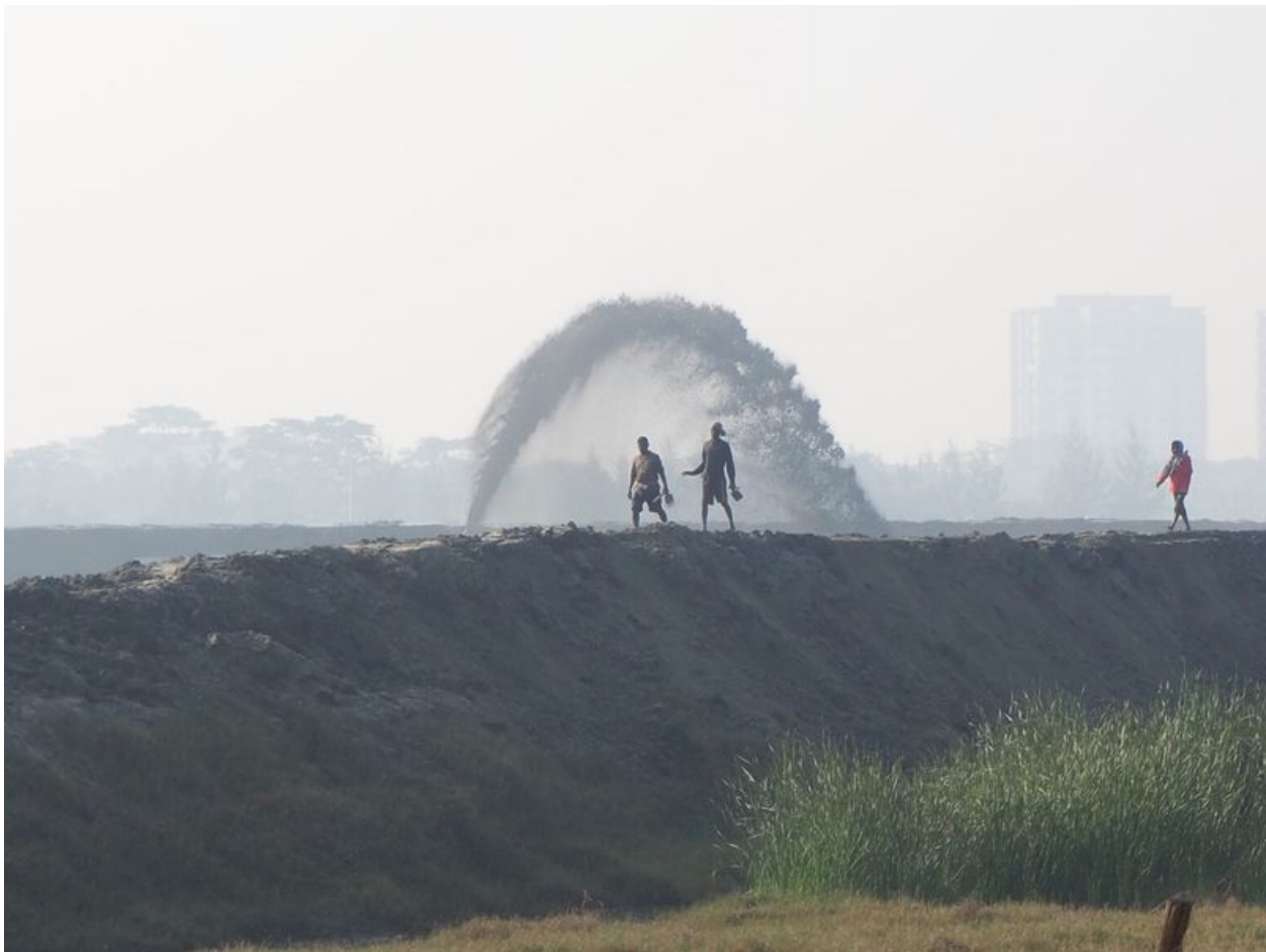
Dredging to build a seawall in Mongla, southwestern Bangladesh, a paradigmatic site of the practice of climate dystopia as a political project. Credit: Jason Cons.
