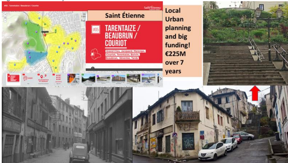
Figure 39: Area disrepair in Saint Étienne
