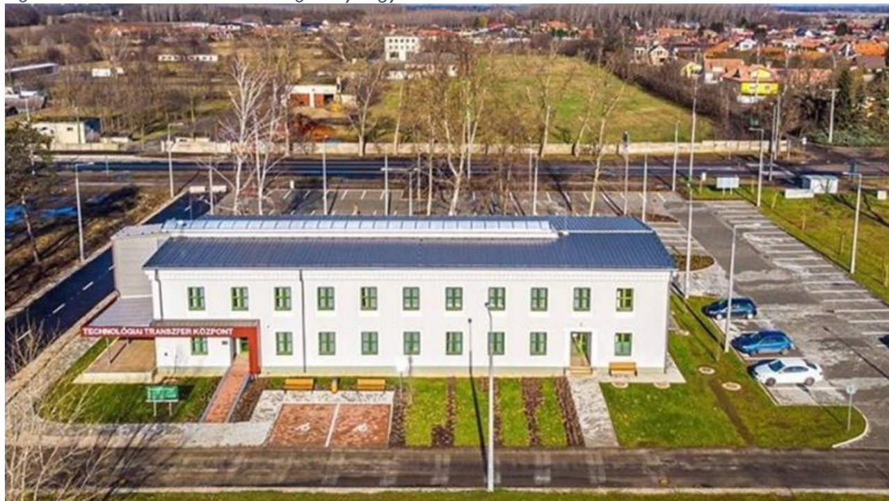
Figure 60: The Incubator Hub building in Nyíregyháza
