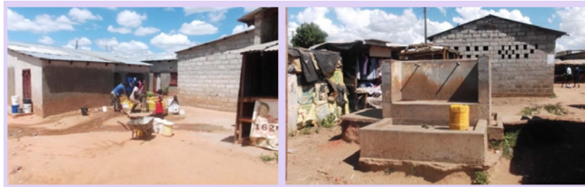
The borehole hand pump constructed during this process. Source: Mwamba, J. S., & Peng, Z. W. (2020). Analysis of Informal Urban Settlement Upgrading: The Case of Ng'ombe Slum Upgrading in Zambia. Current Urban Studies, 8, 509-532. https://doi.org/10.4236/cus.2020.84028
