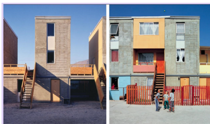
Incremental house, Santiago de Chile, by Elemental (Left: Initial House Delivered. Right: Personalised Houses After Time). Source: Wainer, Ndengeyingoma, and Murray (2016)
