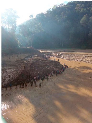
Picture 3 Moving alluvial sand out of the dam reservoir, Taoh Mie District 2017
