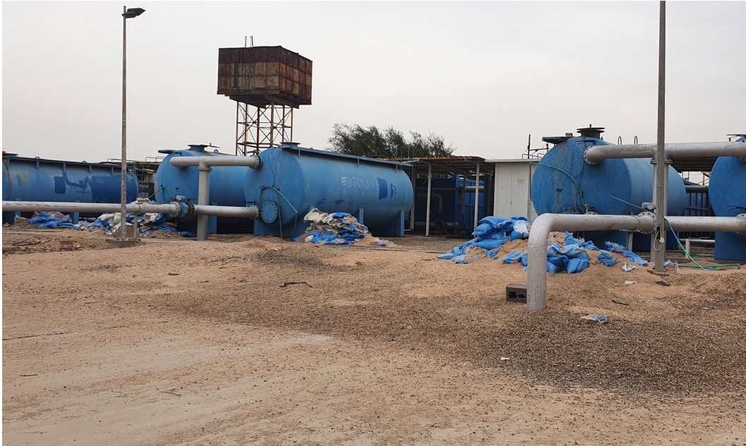
Figure 7: Al Zubayr Water Treatment Plant, November 2020
