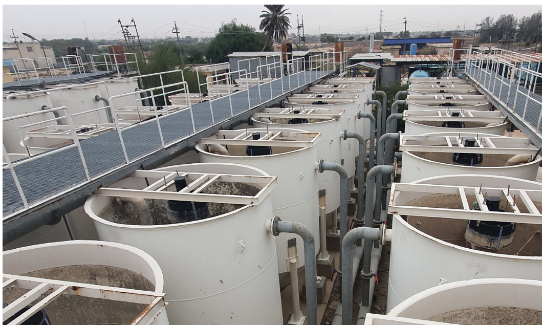
Figure 6: Al Zubayr Water Treatment Plant, November 2020
