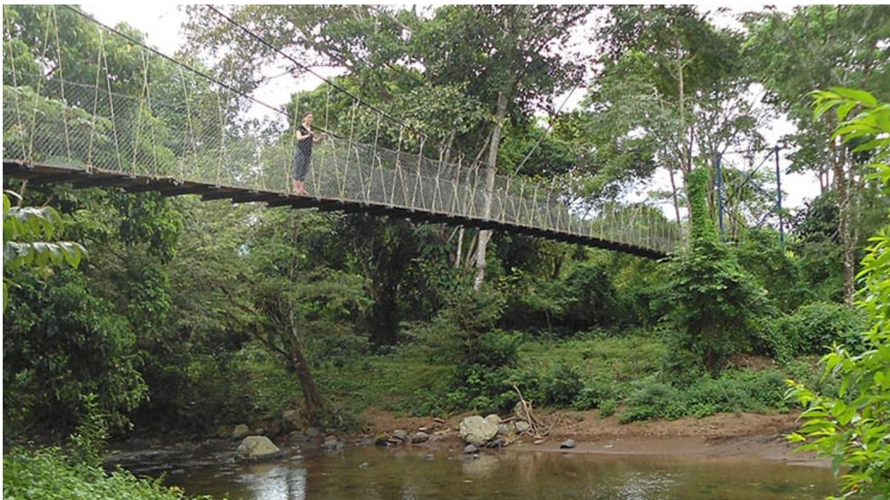
This safe and resilient B2P bridge sits high above a non-flooded riverbed, but note that the high water mark is approximately a metre and a half back from the water's edge and roughly a metre higher (© 2021, Kevin Donovan)
