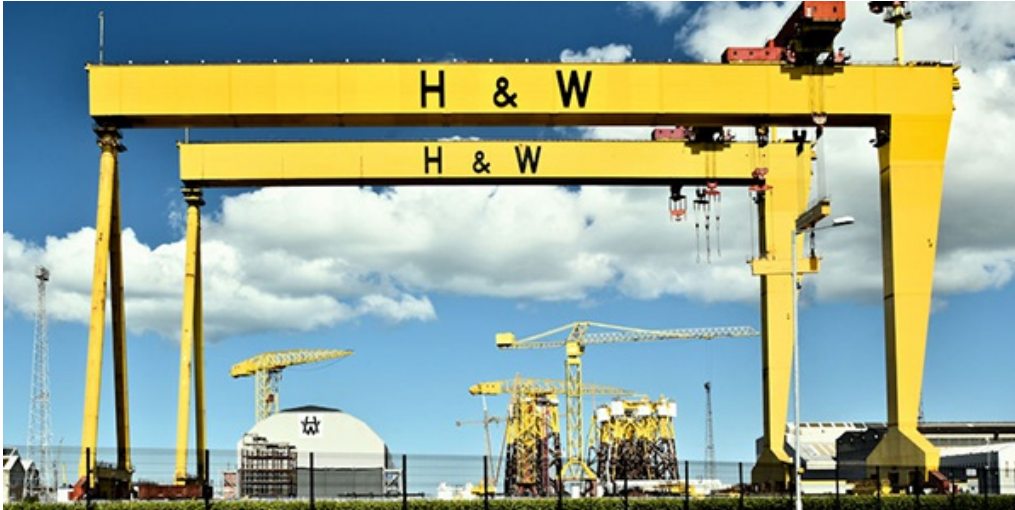
Harland & Wolff cranes, Belfast (May 2019). Picture: Albert Bridge, via geograph.ie/(CC BY-SA 2.0) licence
