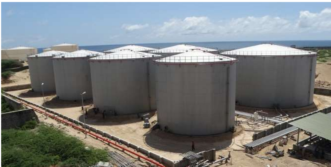
Oil storage facilities in Mogadishu. Source: Joakim Gundel.
