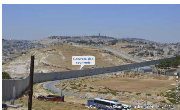
(a) Concrete barrier
